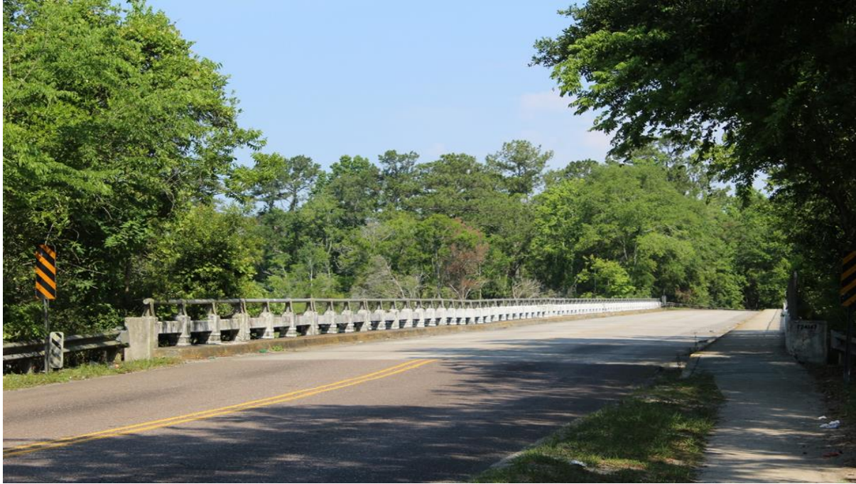
Ribault River Bridge, pre-construction
